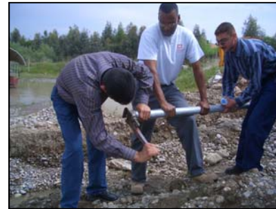
Installing orifice line
