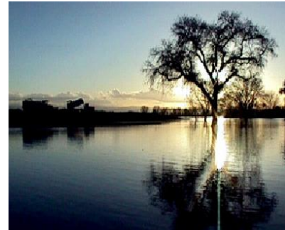
Levee system in Manteca, CA. FEMA photo by Dave Gatley
