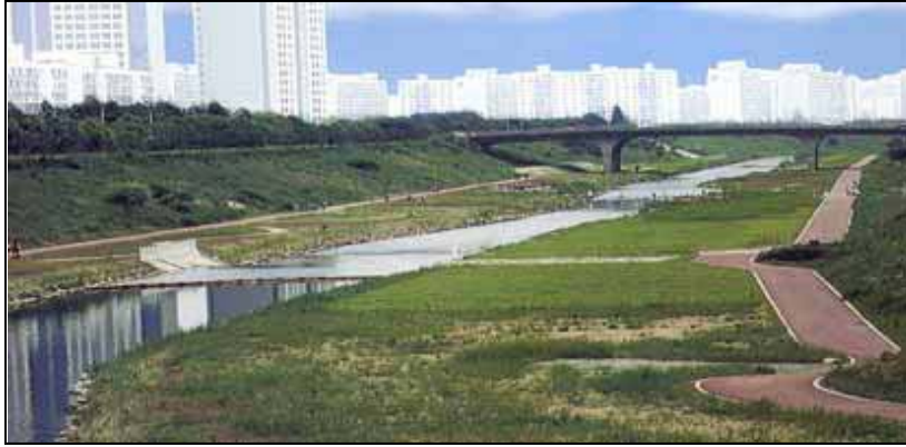
Yangjae-cheon (stream) Restoration Project Site, Seoul, South Korea
