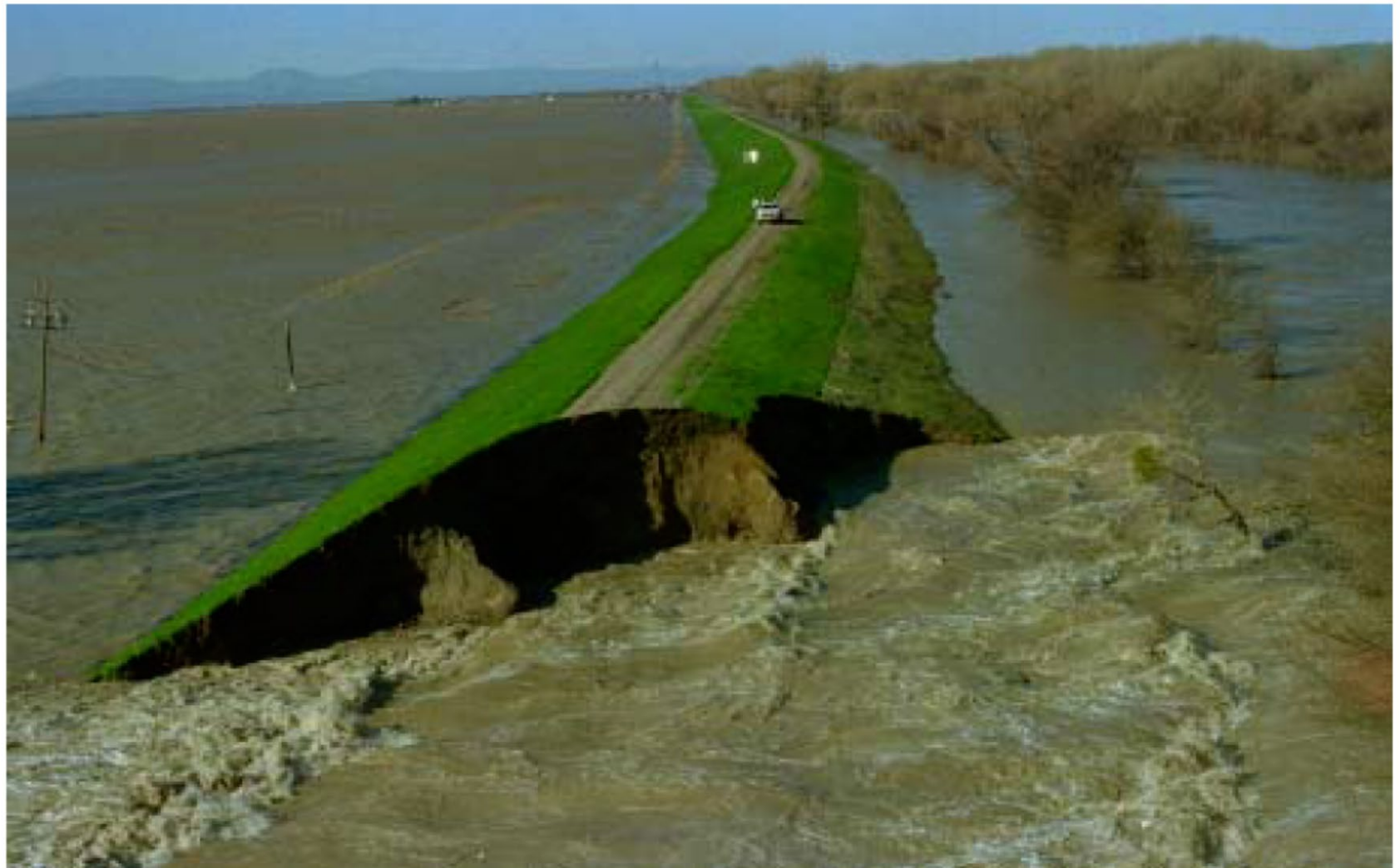
Unanticipated Failure of Sutter Bypass Levee in the 1997 Floods.
