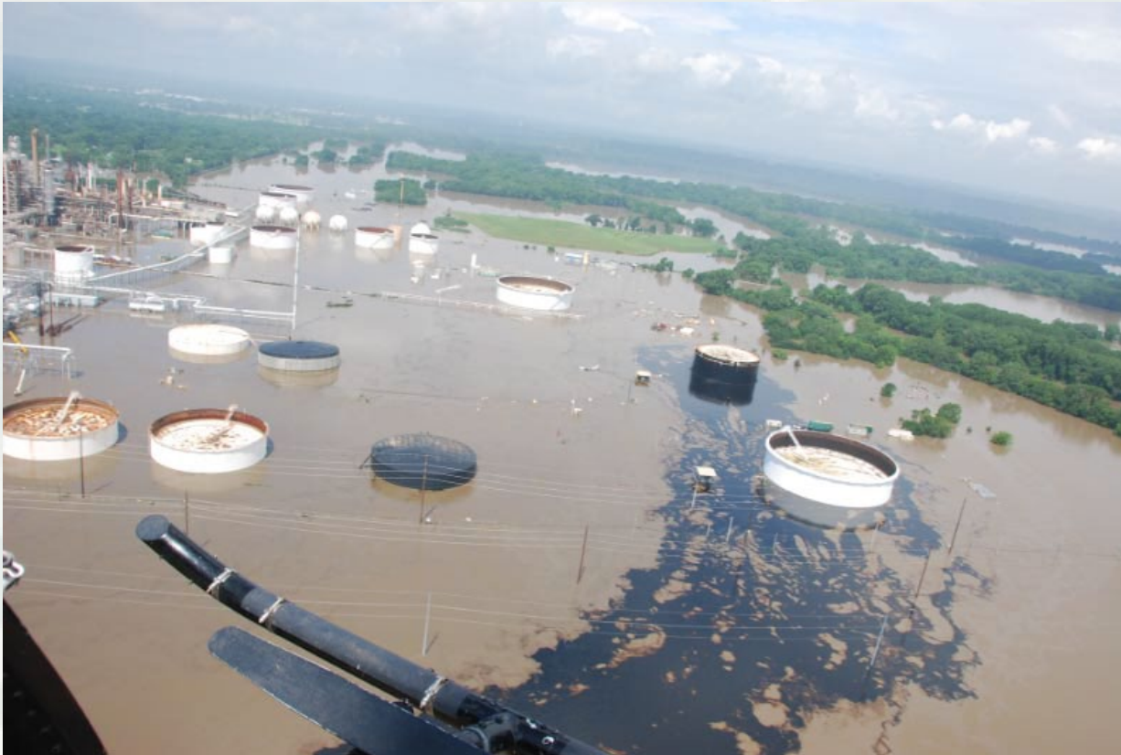
Riverine floodwaters moved one storage tank off its foundation and caused leaking in other tanks, spilling ~2,145 barrels of crude and diesel oil. Coffeyville, KY 2007
