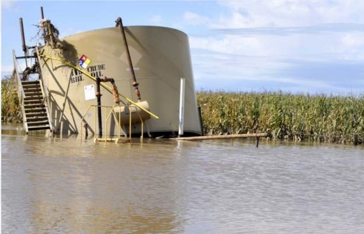
The 2013 Colorado Front Range Flood unseated and toppled several storage tanks, spilling thousands of gallons of crude oil. Weld County, CO 2013
