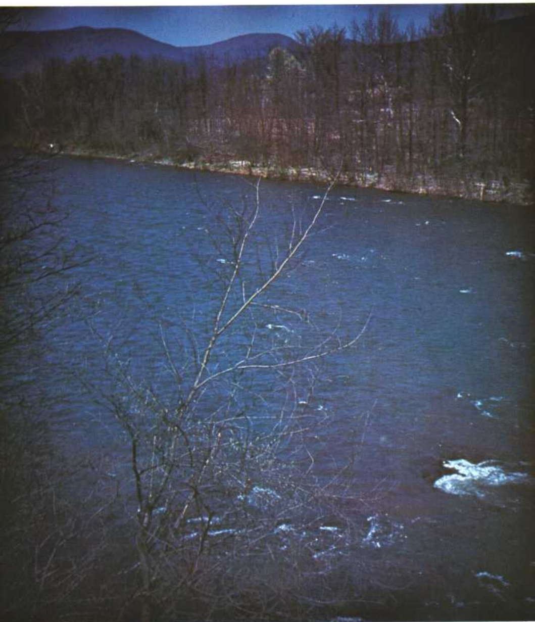
No. 357 upstream from right end of bridge below reach, Esopus Creek at Coldbrook, N.Y. (at Highway 28-A).
