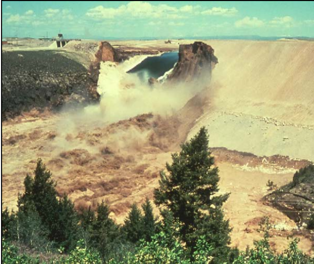
Figure 16. Significant Turbulence and Sediment Load during the Teton Dam Failure (Olsen, 1976)
