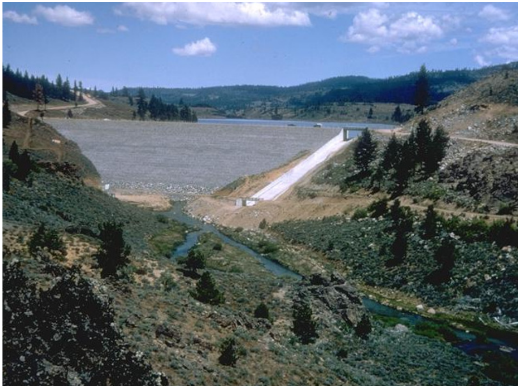
Figure 41. Photograph of dam and spillway (courtesy of California Department of Water Resources)
