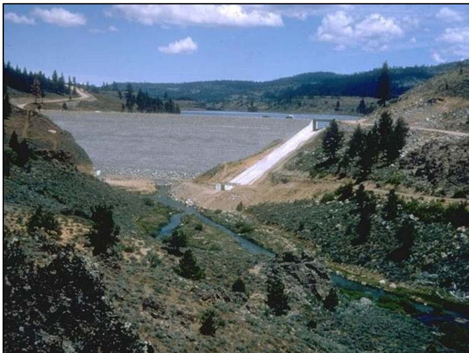
Figure 41. Photograph of Bonanza Dam and Spillway (courtesy of California Department of Water Resources)
