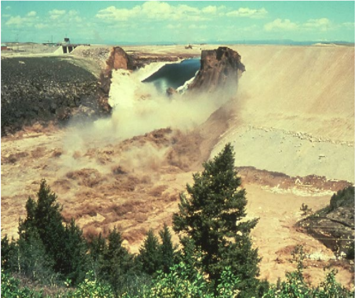
Figure 13-16. Significant Turbulence and Sediment load during the Teton Dam Failure
