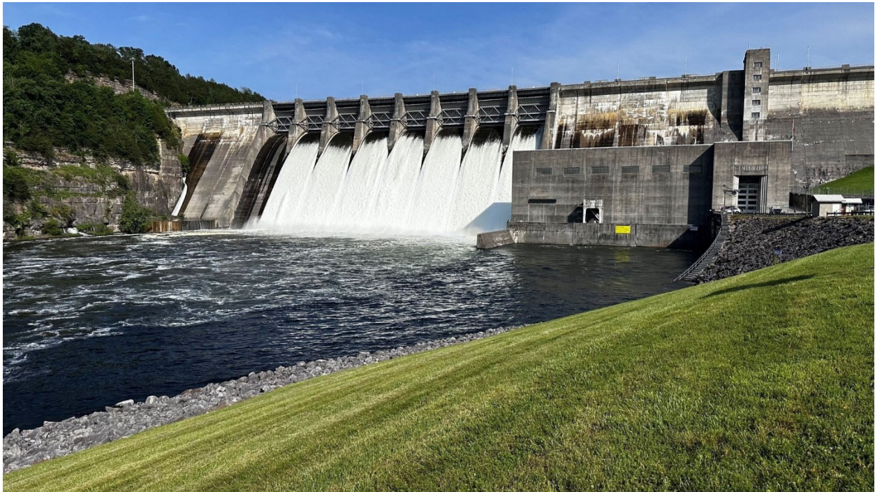
Caney Fork River and Center Hill Dam (USACE photo)
