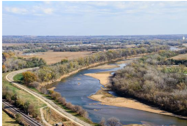
Figure 1. Kansas River, 2021 (USACE photo)
