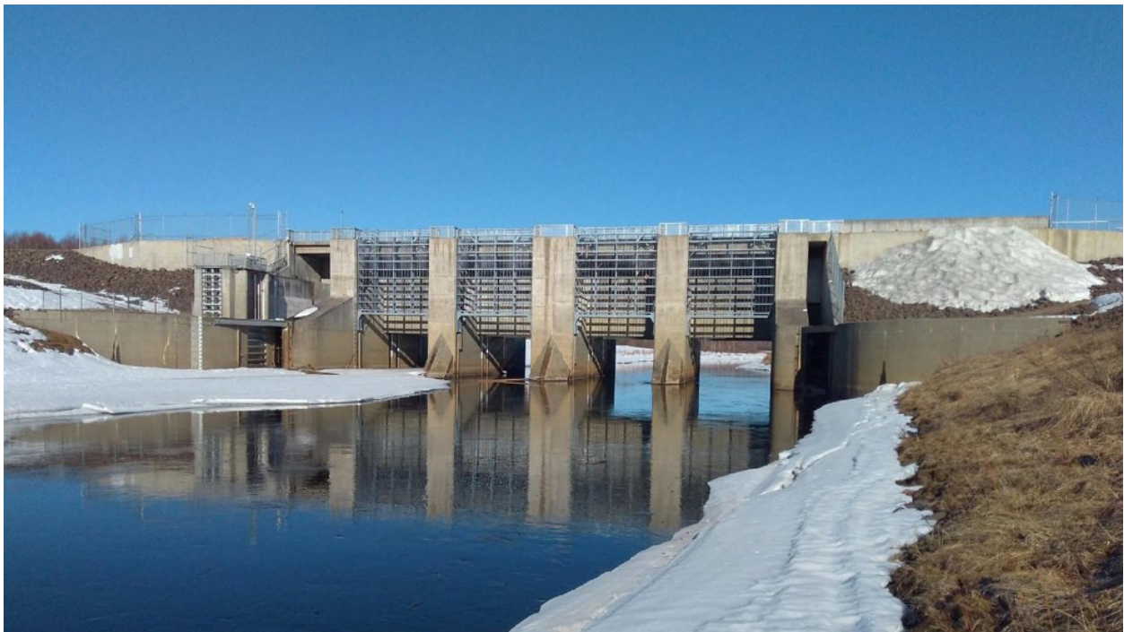
Moose Creek Dam (USACE Photo)
