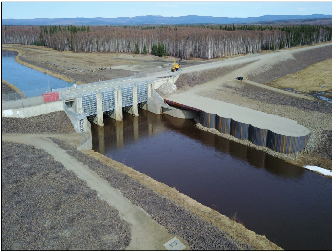
Figure 7. Photo of Moose Creek Dam and its outlet works (USACE photo).
